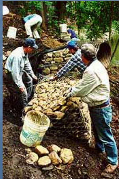
Trail restoration and renovation
